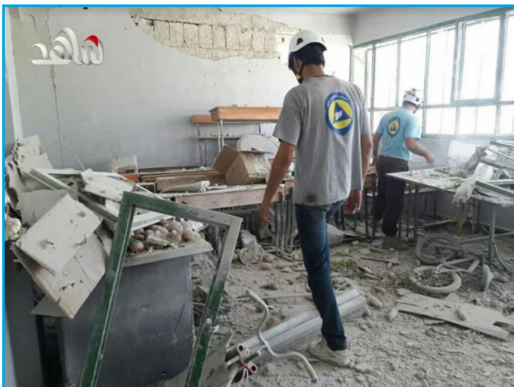
Damages in the aftermath of a bombing by fixed-wing Syrian regime warplanes on the Martyr Yousef Kiwan School in Tafas city, Daraa – June 14, 2017
