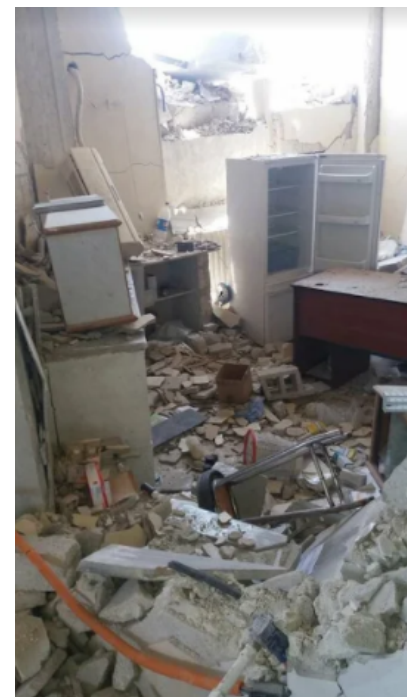
Destruction in Kafr Zita Specialist Hospital inflicted in an attack by fixed-wing warplanes that we believe were Russian – Kafr Zita, Hama – March 12, 2018
